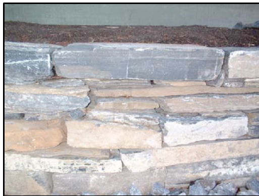
Matherite drystack planter wall detail
