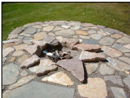
Matherite patio paving with raised rose quartzite
