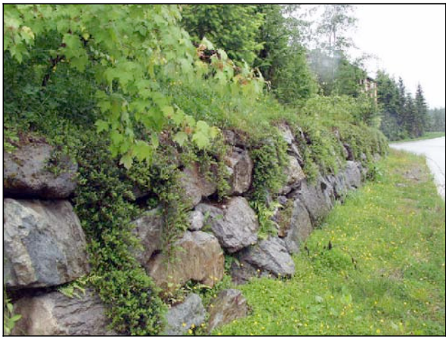
Native Kinnickinnick planting on a roadside retaining wall
