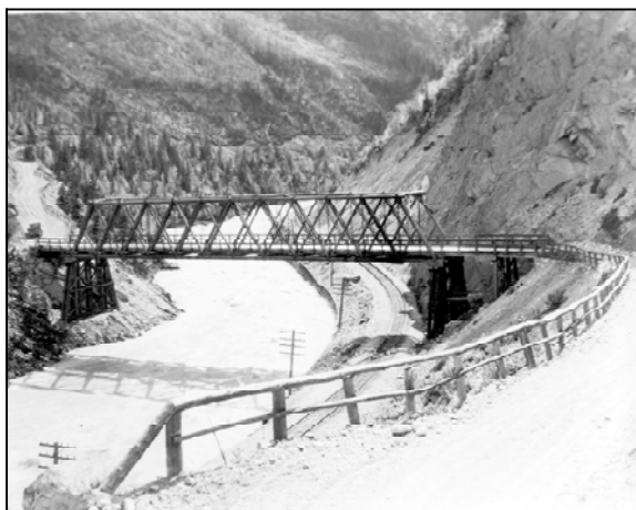
Early road construction - wood guardrail
