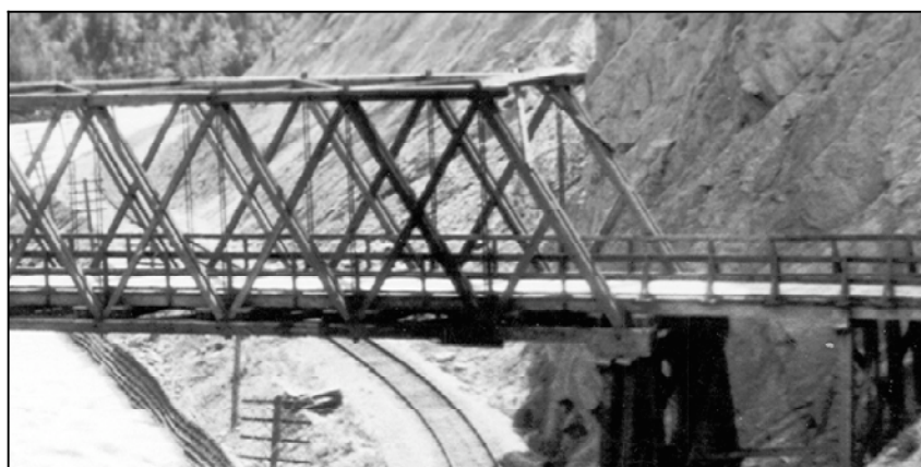
Close-up of trestle construction
